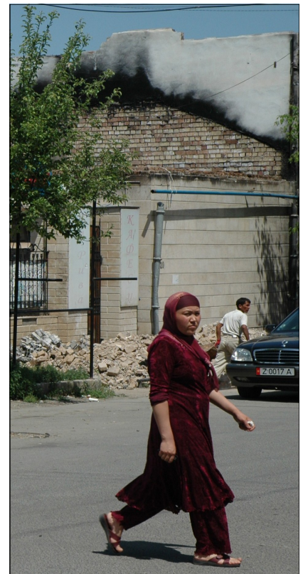
Smoke charred building and rubble still waiting to be cleared
